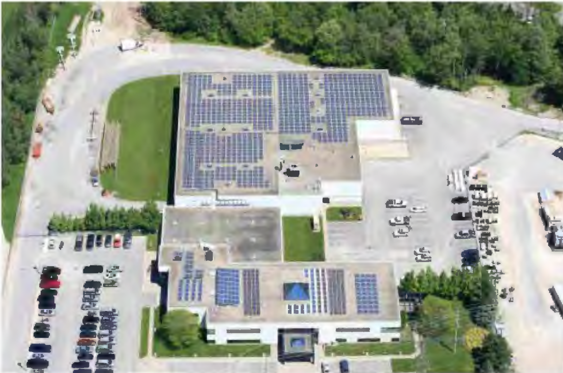
PowerStream's North Operations/Administration Centre in Barrie features a solar PV generation laboratory comprising nine different systems on the roof of the building.
