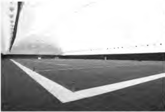
Typical air supported bubble
