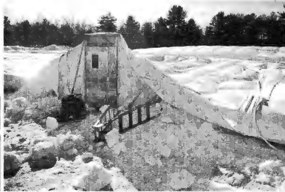
Collapsed bubble due to snow load in Cape Breton
