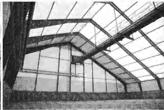
Pre-engineered fabric structure (Legacy-type)
