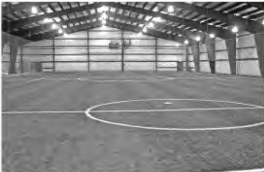
Pre-engineered metal structure
