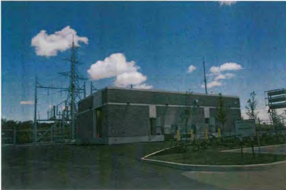
Construction of the Fabro Transformer Station in Markham was completed early in 2010. It is one of 11 transformer stations owned by PowerStream that are directly connected to the provincial transmission grid.
