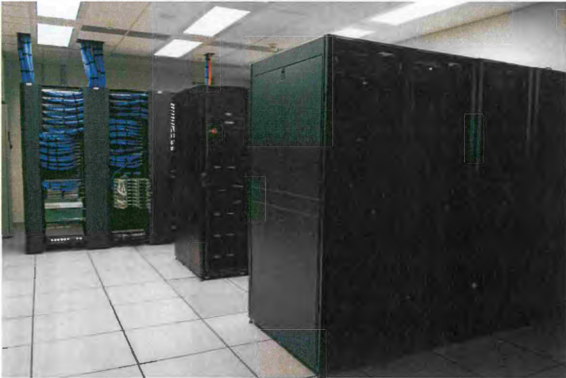
The main data centre at PowerStream's head office in Vaughan connects to the company's two operations centre through fibre optic technology.
