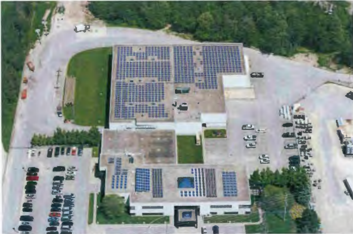
PowerStream's North Operations/Administration Centre in Barrie features a solar PV generation laboratory comprising nine different systems on the roof of the building.
